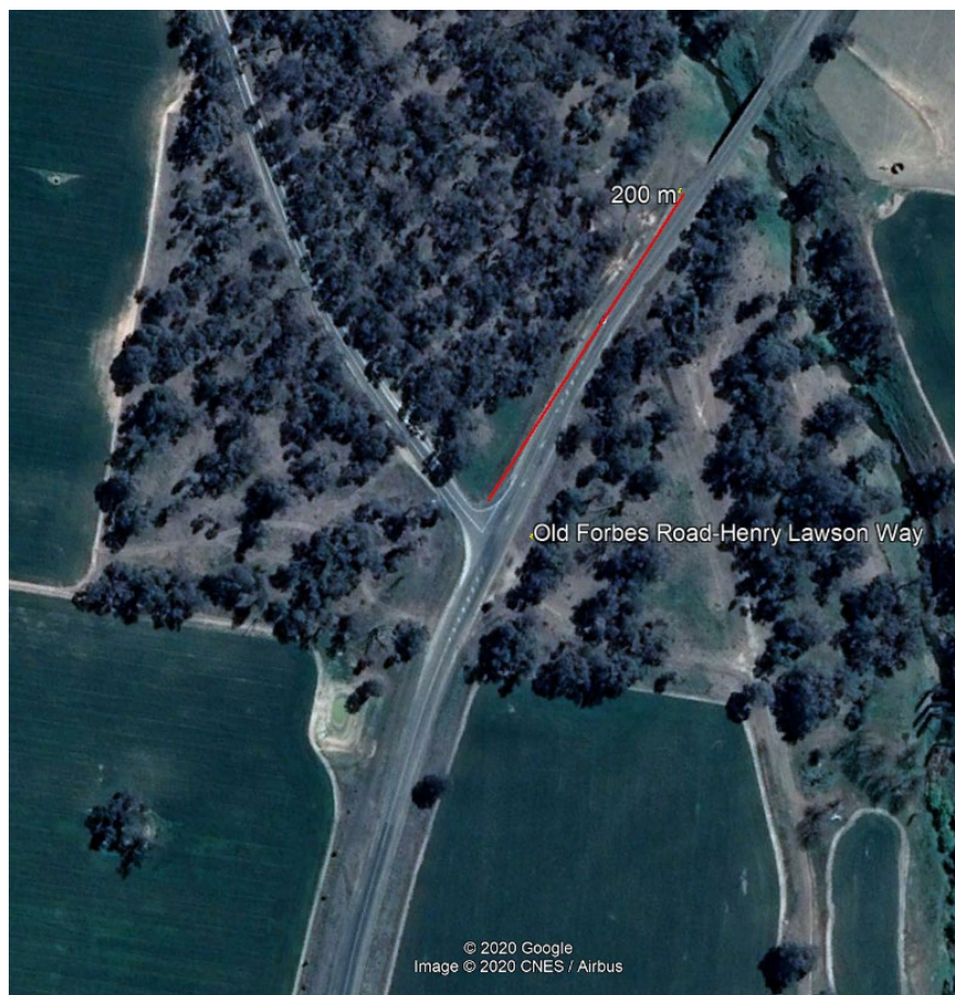
Figure 19 – Junction of Old Forbes Road and Henry Lawson Way
