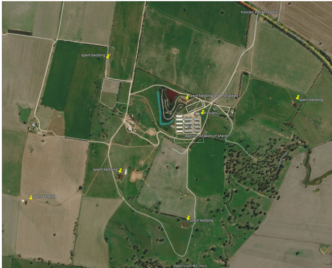
Figure 14 – Spent Bedding Storage Pads
